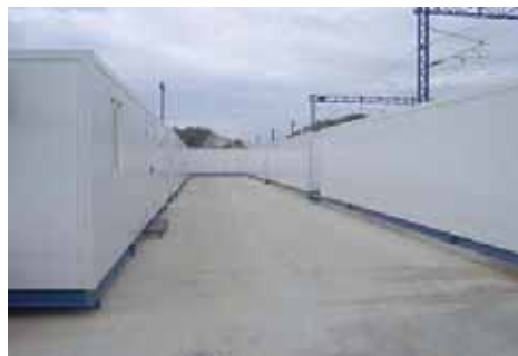
Platform of the Talgo (left) and CAF (right) changers. On the left, a vertically folding platform. On the right, huts for the portable third generation changers
