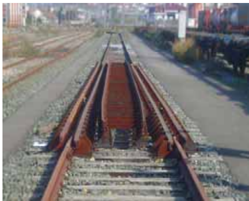
Changer for Rafil and SUV-2000 technologies installed at Irún for tests
