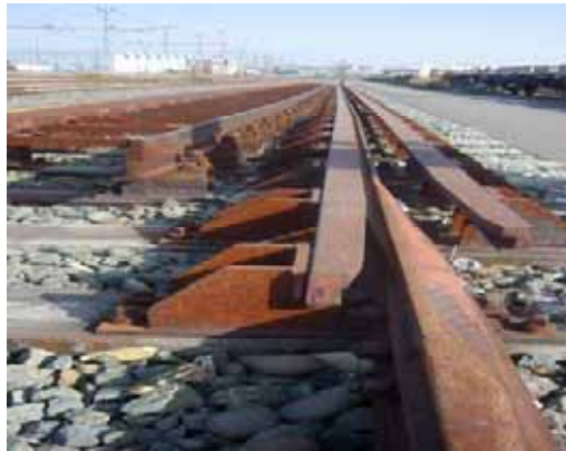
Changer for Rafil and SUV-2000 technologies installed at Irún for tests
