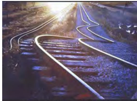
Meckering (WA) Earthquake, 14th October 1968 ( Photo courtesy of Alice Snooke)
