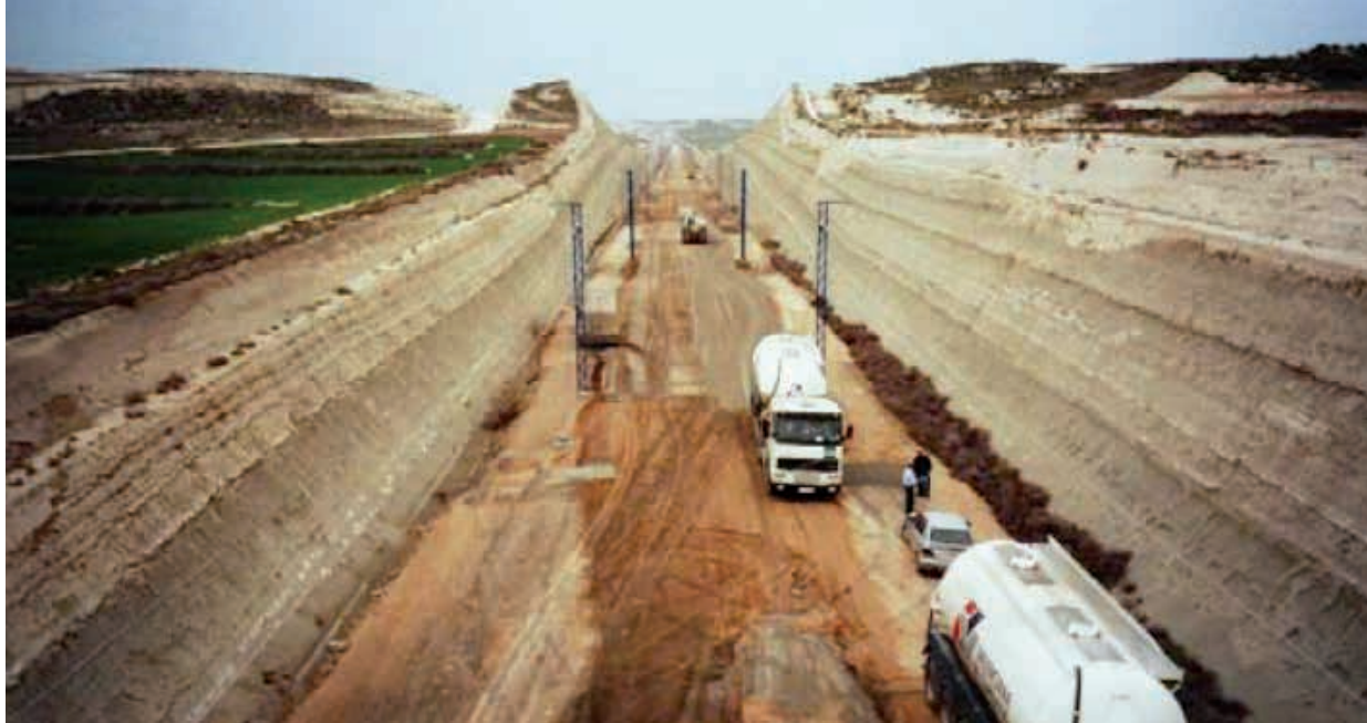
Photo 3 Stabilizing the platform in Zaragoza
