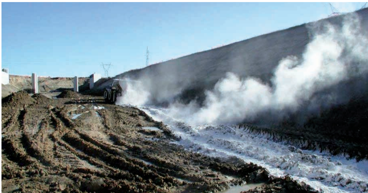
Photo 2 Drying the platform in Olmedo
