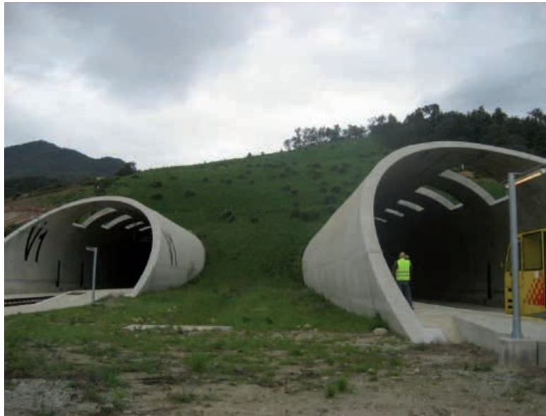
Figure 6. North Porous Portal. Perthus Tunnel.
