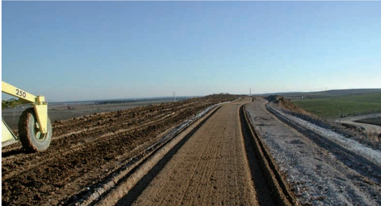
Photo 1 Drying the platform
