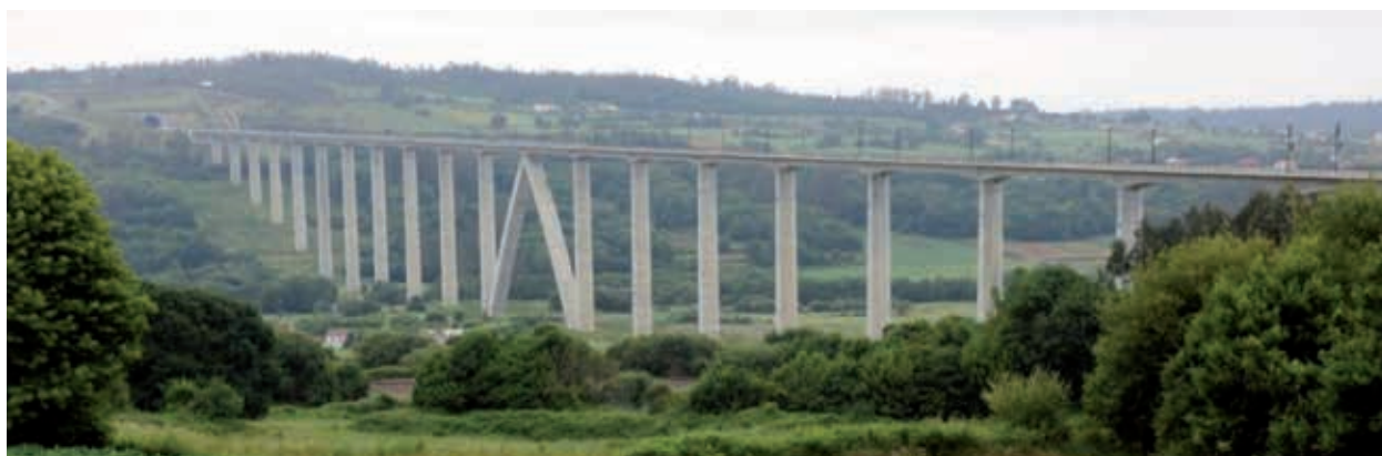
Figure 2. O Eixo Viaduct in the High-speed line Madrid - Galicia
