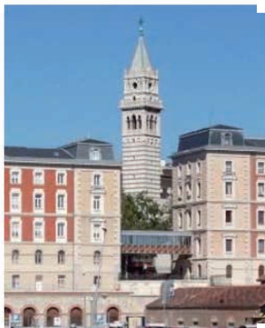
Figure 50: Old MZA offices and Pantheon's campanile. Source: Juan Ayrault
