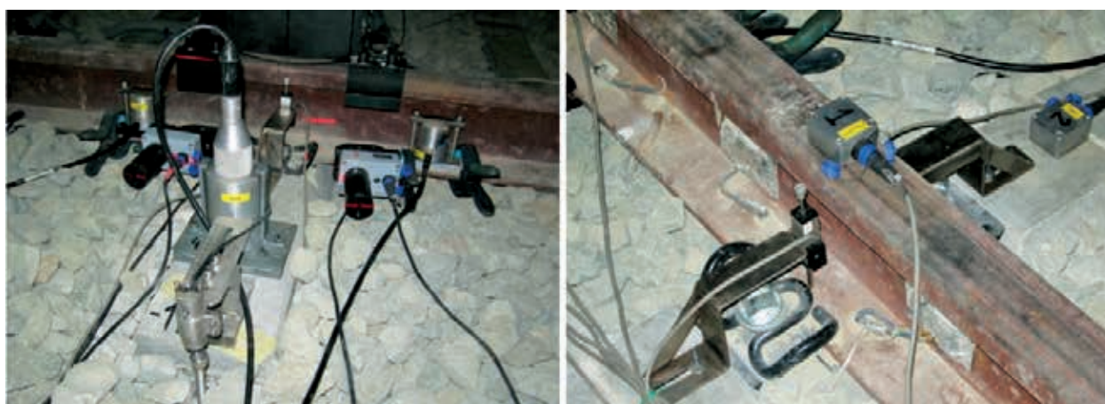
Figure 3. View of some of the instrumentation installed in the superstructure
